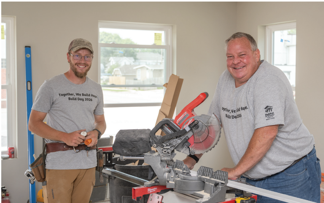
Logan Erickson (Master Carpenter) from Erickson Carpentry & Robin Debe (Founder) from Realistic Builders are prepping trim for installation.
