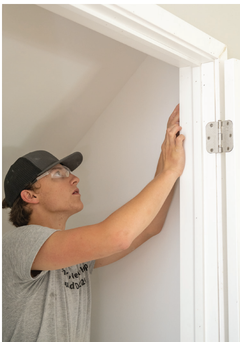
Adam Langendorf (Project Manager) from Realistic Builders, completes interior trim of the pantry door.
