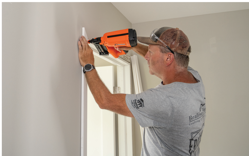
Jeff Erickson (Master Carpenter/Owner) from Erickson Carpentry is installing door trim for the upstairs bedroom.
